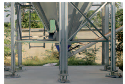
Silo scale with electronic load cells
