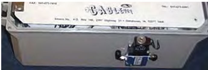
Photo #5 - Air Valve
