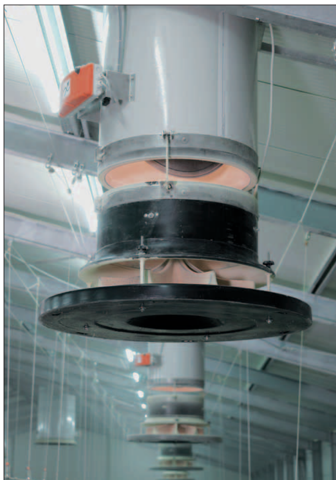
Fumus fresh air chimney for equal or positive pressure ventilation
