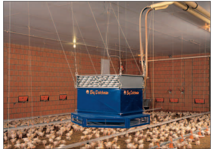
Implementation of HEAT MASTER 40 in a broiler house
