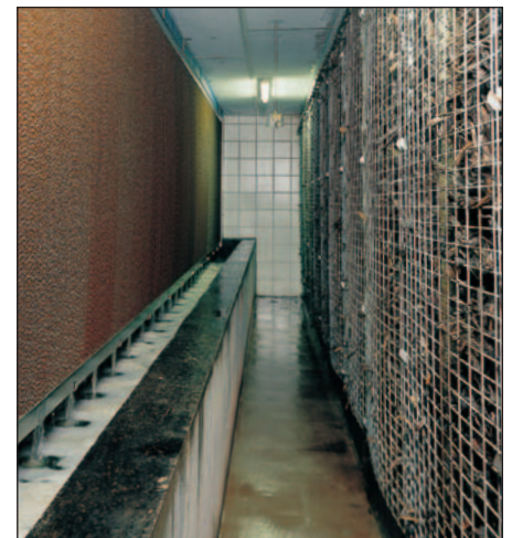
The third treatment step consists of root timber and is used for the microbial transformation of odour-carrying agents.
