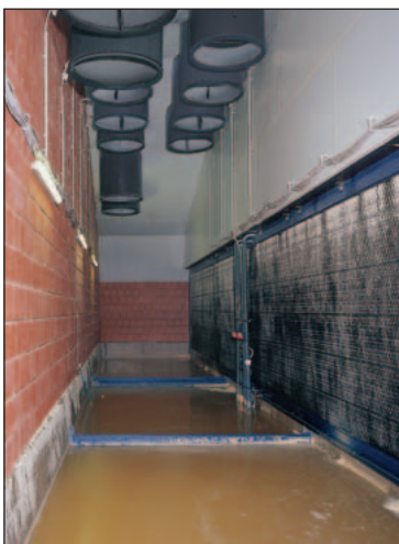
Back view of the filter – exhaust air chimneys suck the house air through the filter –
