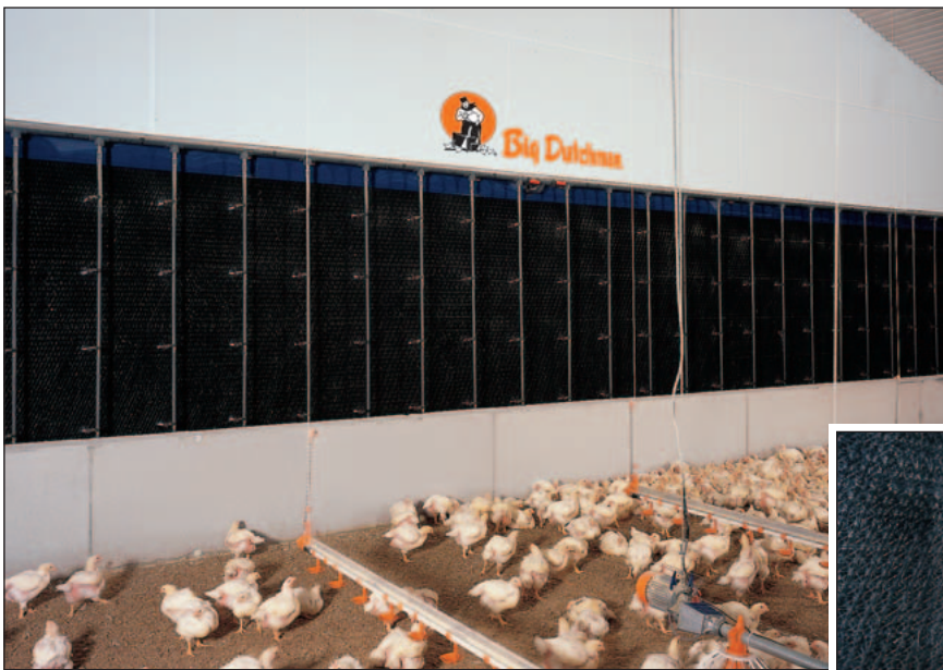
Back view of the filter – exhaust air chimneys suck the house air through the filter –
